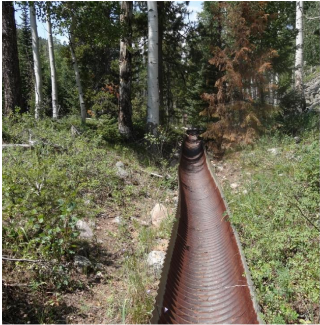
Figure 3: CMHP lined sections of Cedarview Canal. August 5, 2020. (Photos: Brook Watts, Ute Indian Tribe Fish and Wildlife Department)
