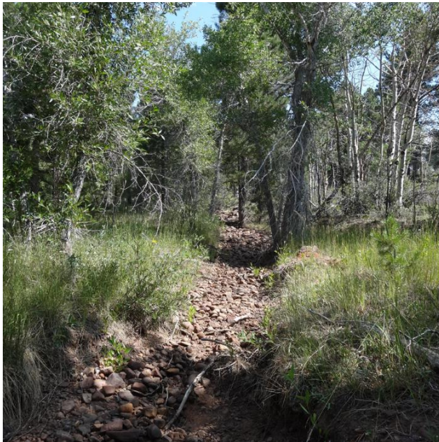
Figure 4: Unlined sections of the Cedarview Canal. August 5, 2020. (Photos: Brook Watts, Ute Indian Tribe Fish and Wildlife Department)
