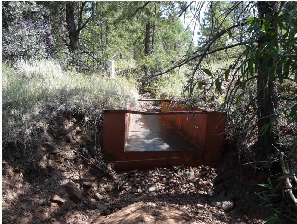
Figure 6: Cutthroat flume and stilling well at the southern end of the Cedarview Canal. August 5, 2020. (Photo: Brook Watts, Ute Indian Tribe Fish and Wildlife Department)
