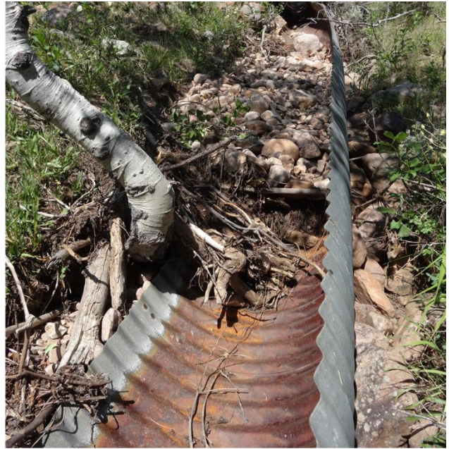
Figure 3: CMHP lined sections of Cedarview Canal. August 5, 2020. (Photos: Brook Watts, Ute Indian Tribe Fish and Wildlife Department)
